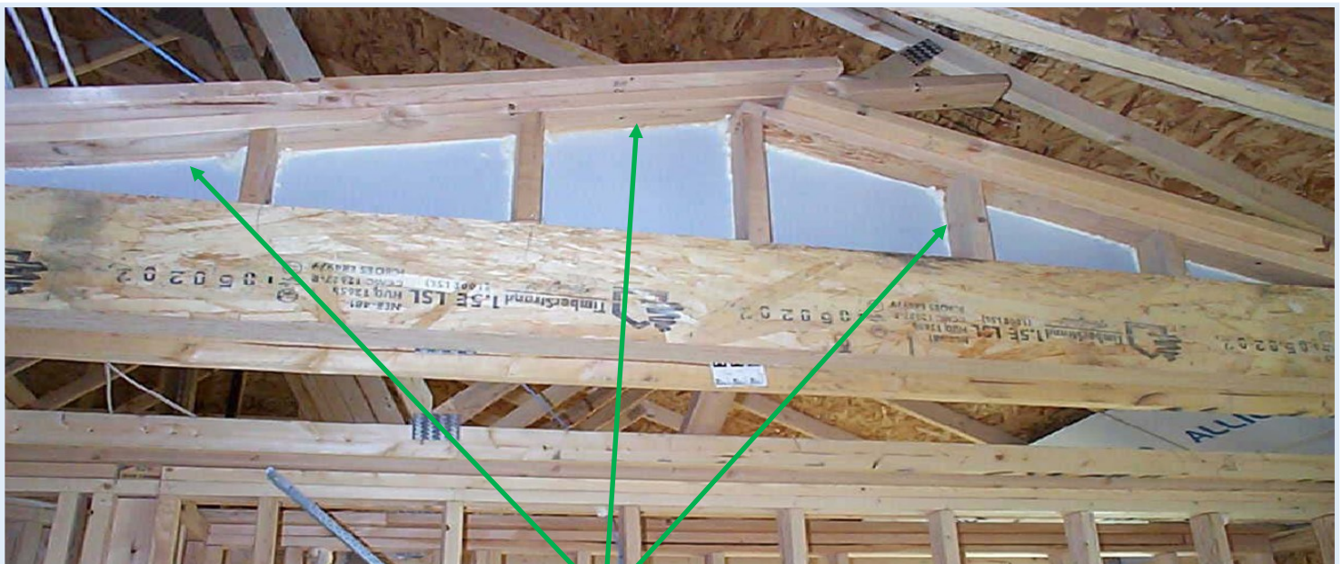
Air sealing at the air barrier for the attic knee wall
