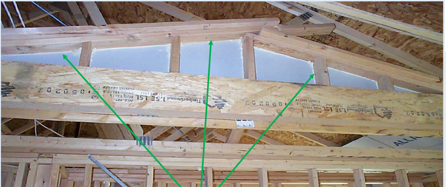
Sealing provided at bottom (sill) plate and at top plate
