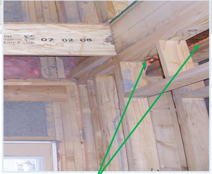
Sealing provided at bottom (sill) plate and at top plate
