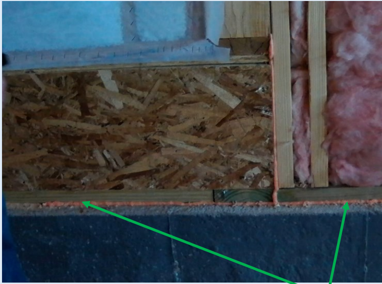
Sealing provided at bottom (sill) plate and at top plate
