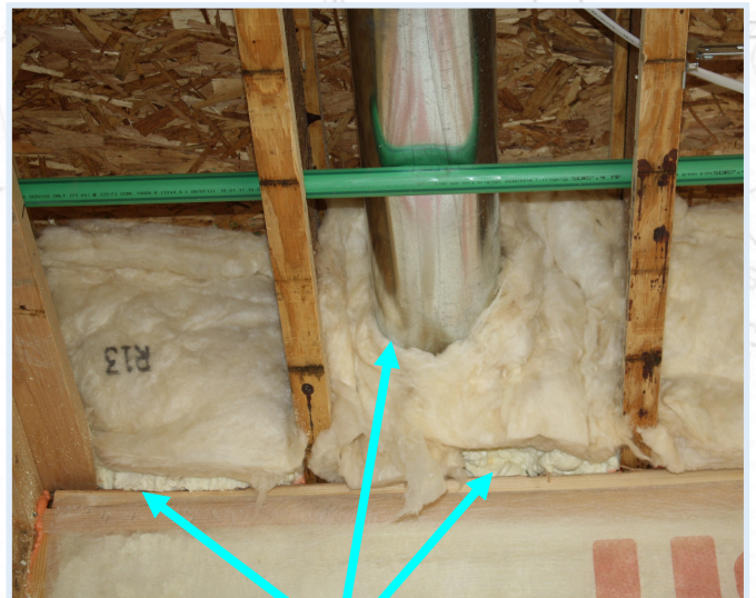
Exhaust duct sealed by the spray foam used in the rim joist because it meets or exceeds the required thickness to be an air barrier.
