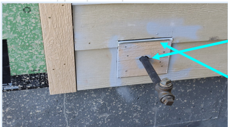
This gas line utility penetration will need to be air sealed to allow for expansion and contraction.
