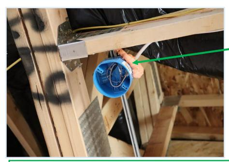
This electrical box is penetrating at the ceiling drywall which is where the thermal envelope and air barrier are located. The wires entering the electrical box have been sealed.
