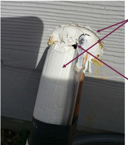
The hole created for this penetration was larger than it needed to be for the penetration. This penetration is an odd-shaped penetration that will require some thought on how to create an air seal which will work and last.
