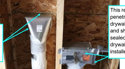
This register will be penetrating the drywalled ceiling, and should be sealed to the drywall when installed.
