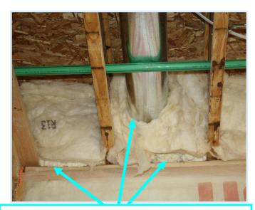
Exhaust duct sealed by the spray foam used in the rim joist because it meets or exceeds the required thickness to be an air barrier.
