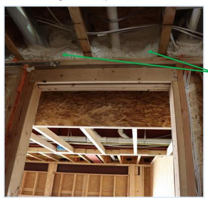
Spray foam to a thickness that includes it to be used as an air barrier. The spray foam was installed on the side of the dwelling unit and not on the side of the garage. It does still separate the garage from the conditioned space.
