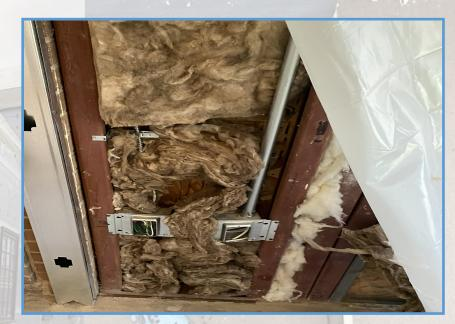
Both of these images demonstrate insulation compressed (crammed into the cavity)
