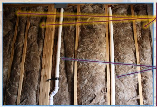
The insulation for this install was compressed in the cavities
