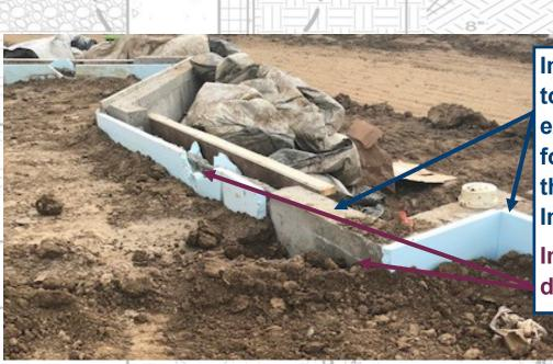
Insulation installed at top of foundation on the exterior side of the foundation and where the slab will be poured. -Intent good
