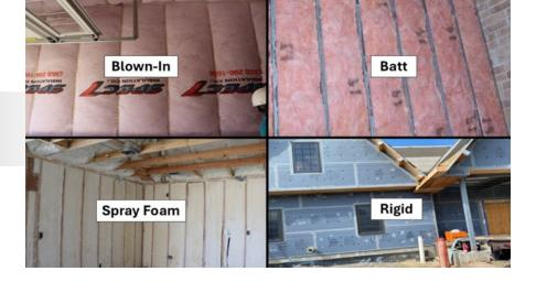
**Purpose:** To identify the different types of insulation, installation methods, uses and thermal resistance.
